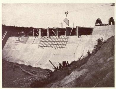
ORK has been concentrated upon the roll-way of the dam and in the past twenty days the buttresses, the deck and the apron have progressed to this stage.
